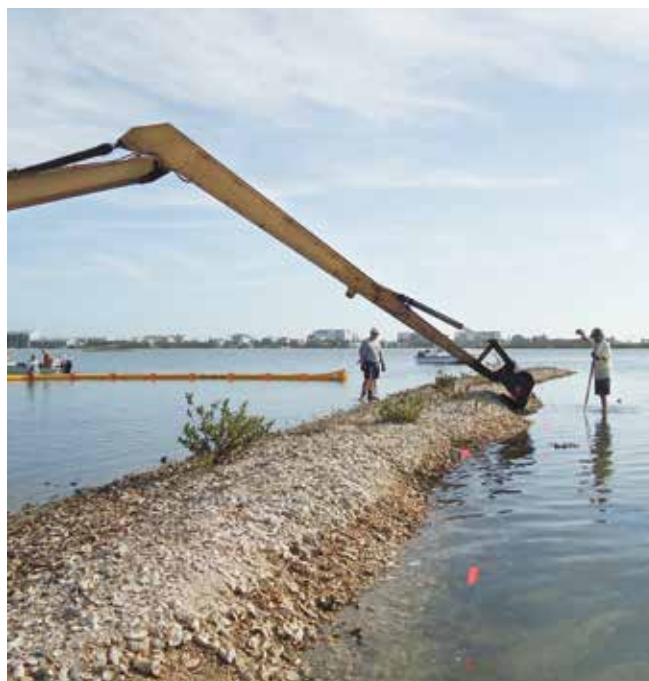
Excavator, Mosquito Lagoon: The overall project goal is to increase the areal coverage of live intertidal oyster reefs by leveling the dead margins and covering the shell material with oyster mats, a stabilized recruitment substrate for oysters. © Anne P. Birch, The Nature Conservancy
