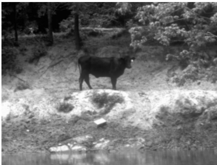
Figure 4. Bank Erosion from Livestock Intrusion.
